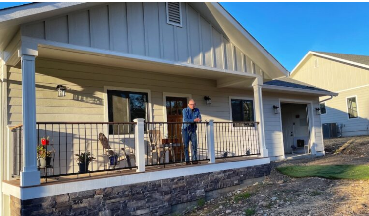
Dick on the porch of the ADU
