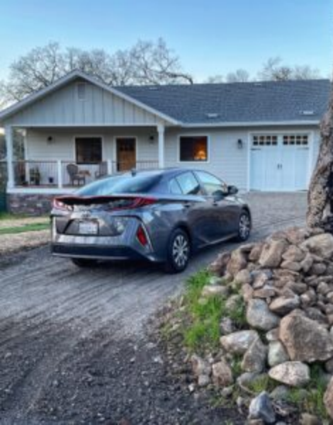
The driveways are still not finished. Since this picture was taken most of the pavers are in place.
