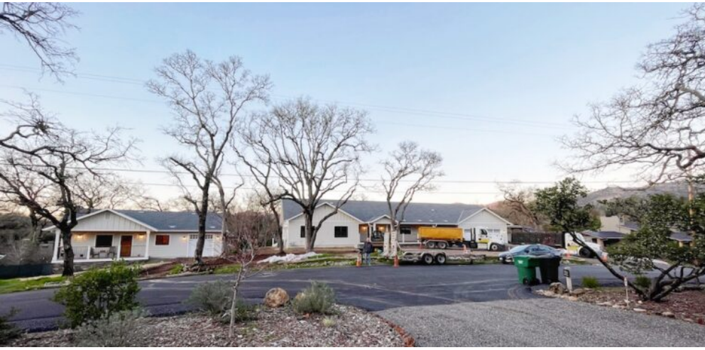
Main house and ADU, mostly finished
