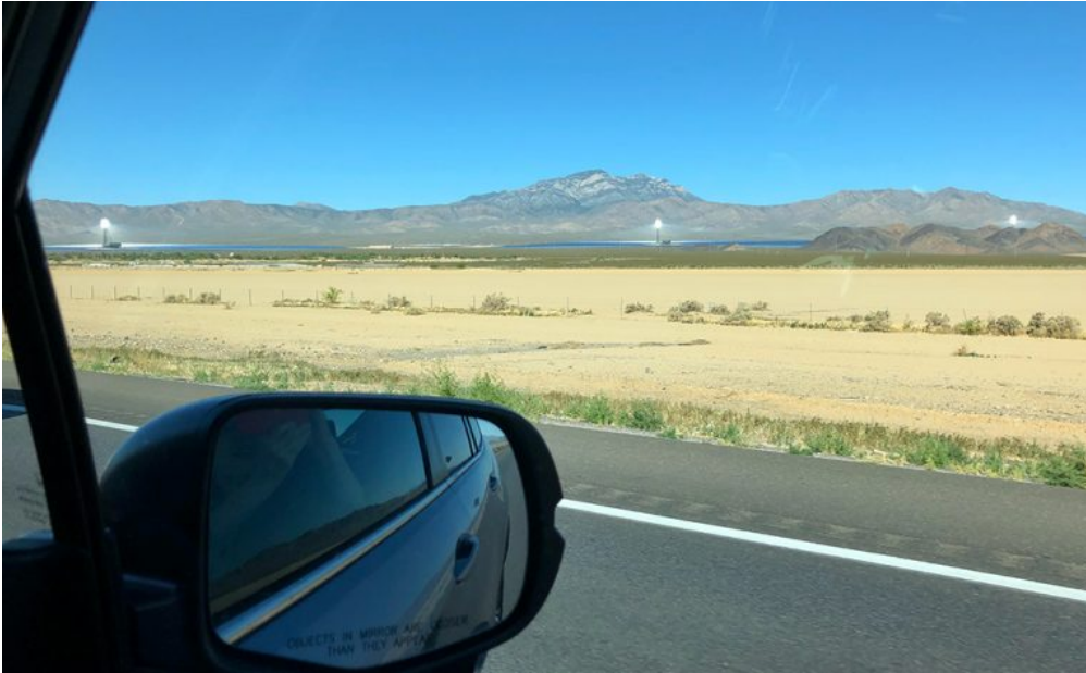
Solar panel and collector farm in the Mojave Desert
