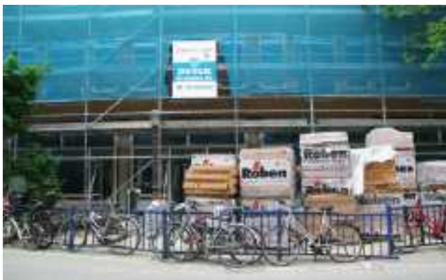
Figure 61: Neighborhood renovation (in 2006)
