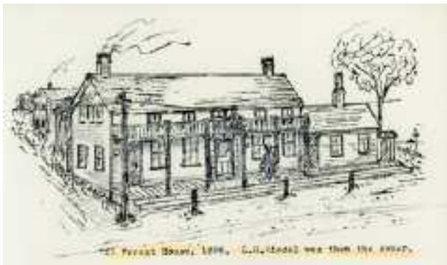
Figure 30: Forest House on the East End (Courtesy Ed Wahla)
