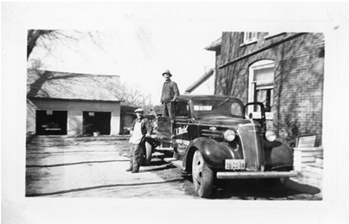
Garage (former barn) behind the Red House
